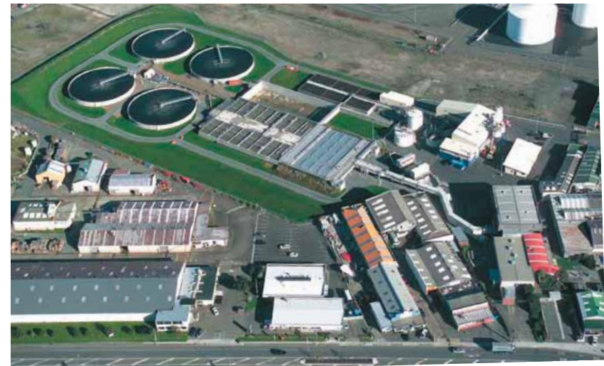
Aerial photograph of the Wastewater Treatment Plant in Seaview
