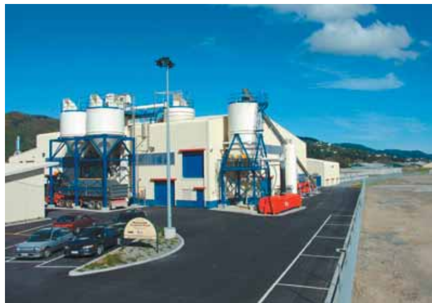
Council's Wastewater Treatment Plant in Seaview
